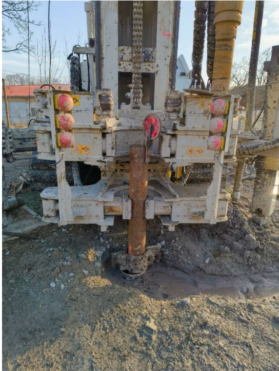
Vrtná souprava – detail
